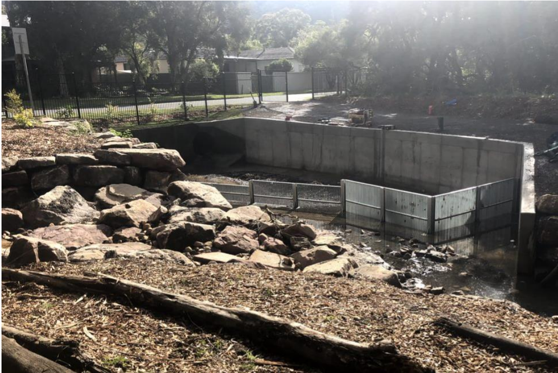
Figure 3: Completed GPT at Wairakei Road, Wamberal
