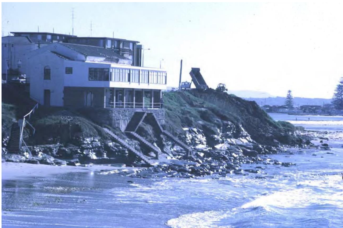
Figure 3-25 South Entrance Beach in 1974 showing the Beach Completely Eroded Away after Extreme Erosion Event(s) (image sourced from Umwelt, 2011a)
