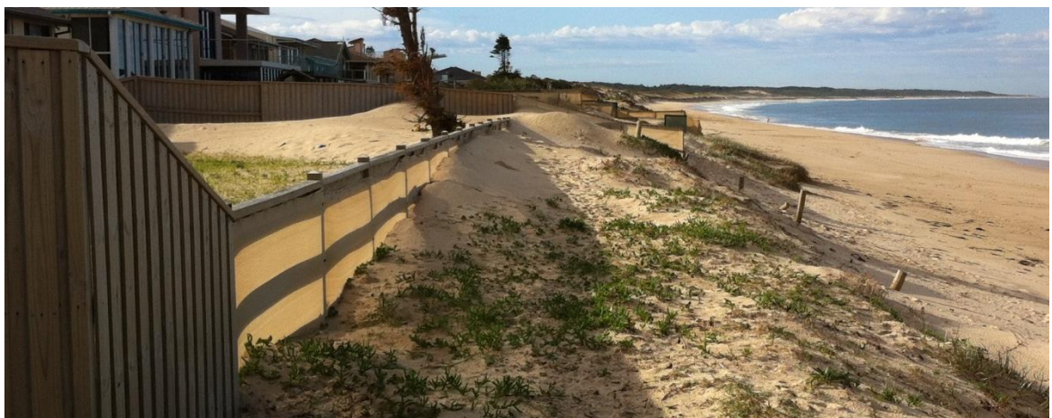
Figure 3-27 Tuggerah Beach Compartment, looking north from North Entrance Beach (Curtis Parade); note the Sand Drift and Proximity of the Houses to the Foreshore
