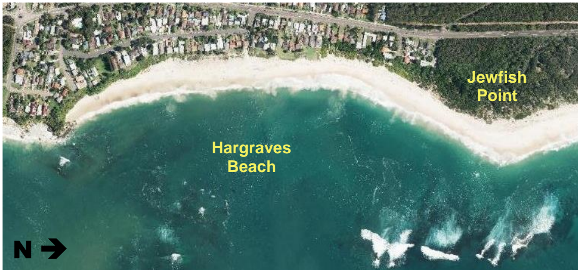
Figure 3-52 Aerial Image of Hargraves Beach, showing the Two Offshore Reefs and Their Control on the Beach Form (e.g. Jew Fish Point); Note the Proximity of Residential Development to the Foreshore in the Middle Section of Beach
