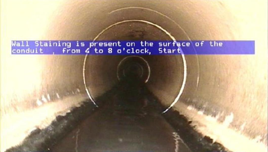
Wall Staining is present on the surface of the conduit , from 4 to 8 o'clock, Start
