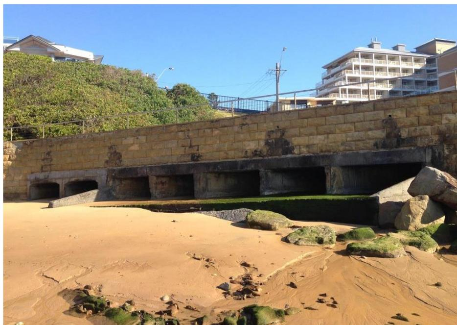
Figure 6: Large stormwater culverts where the majority of stormwater from the catchment exits onto Terrigal Beach.
