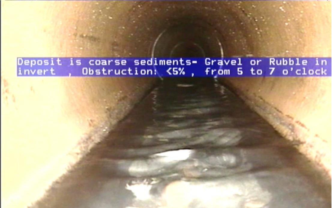
Deposit is coarse sediments- Gravel or Rubble in invert , Obstruction: <5% , from 5 to 7 o'clock
