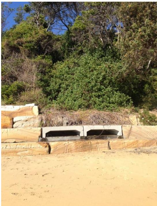
Figure 9: Eastern stormwater culverts entering Terrigal Haven Beach from Scenic highway and residential areas.
