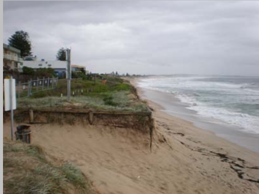
Photo 3 - 8 th February 2008 – severely eroded beach profile
