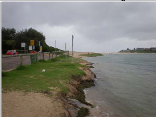
Photo 11 - 8 th February 2008 – severely eroded beach profile
