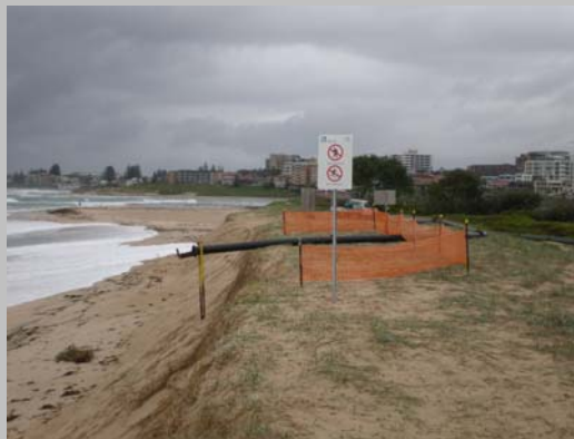
Photo 6 - 8 th February 2008 – severely eroded beach profile with pipeline discharge prepared for beach nourishment activities
