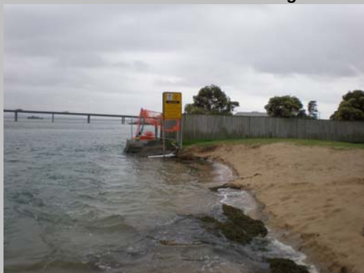
Photo 9 - 8 th February 2008 – severely eroded beach profile – view west from Karagi Foreshore Park towards Dunleith Caravan Foreshore Park
