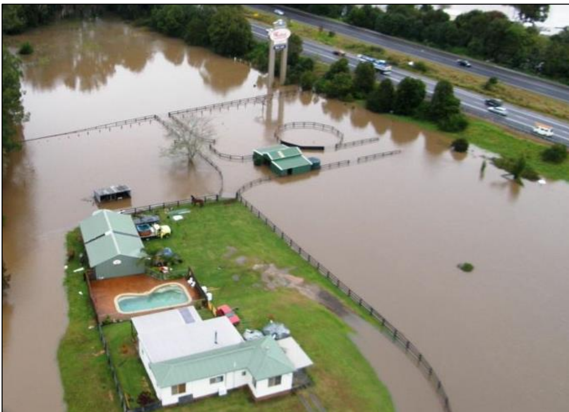
Plate 3 Looking south west from Mardi Road towards Pacific Motorway during 2007 flood (photo provided by the SES via Central Coast Council)
