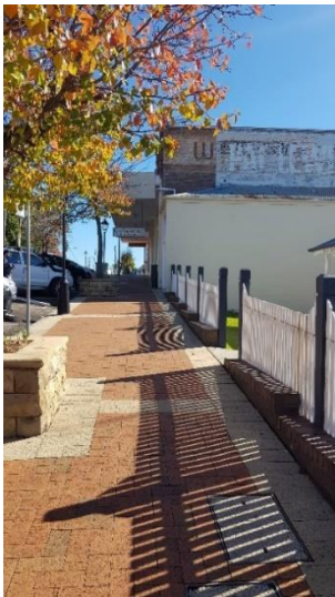
Street Stall Area 1 – Front of Business, - 12 Alison Road Wyang
