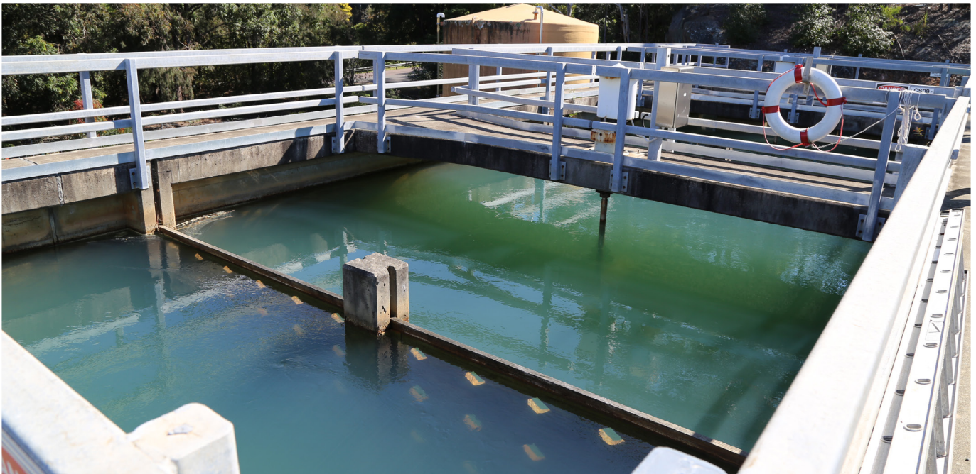
Mardi Treatment Plant - Flocculation Chamber
