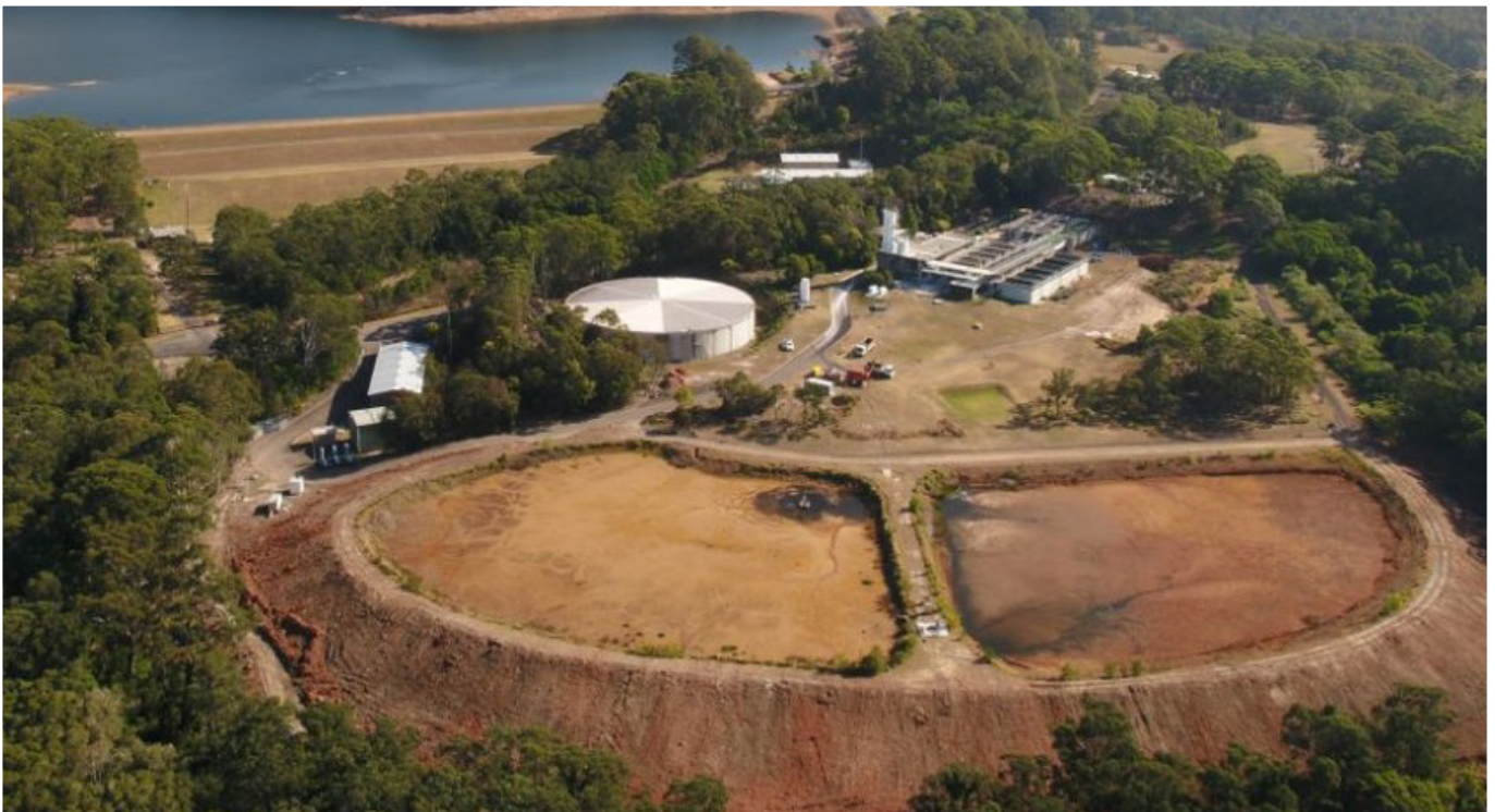
Mardi Treatment Plant - Sludge Lagoons
