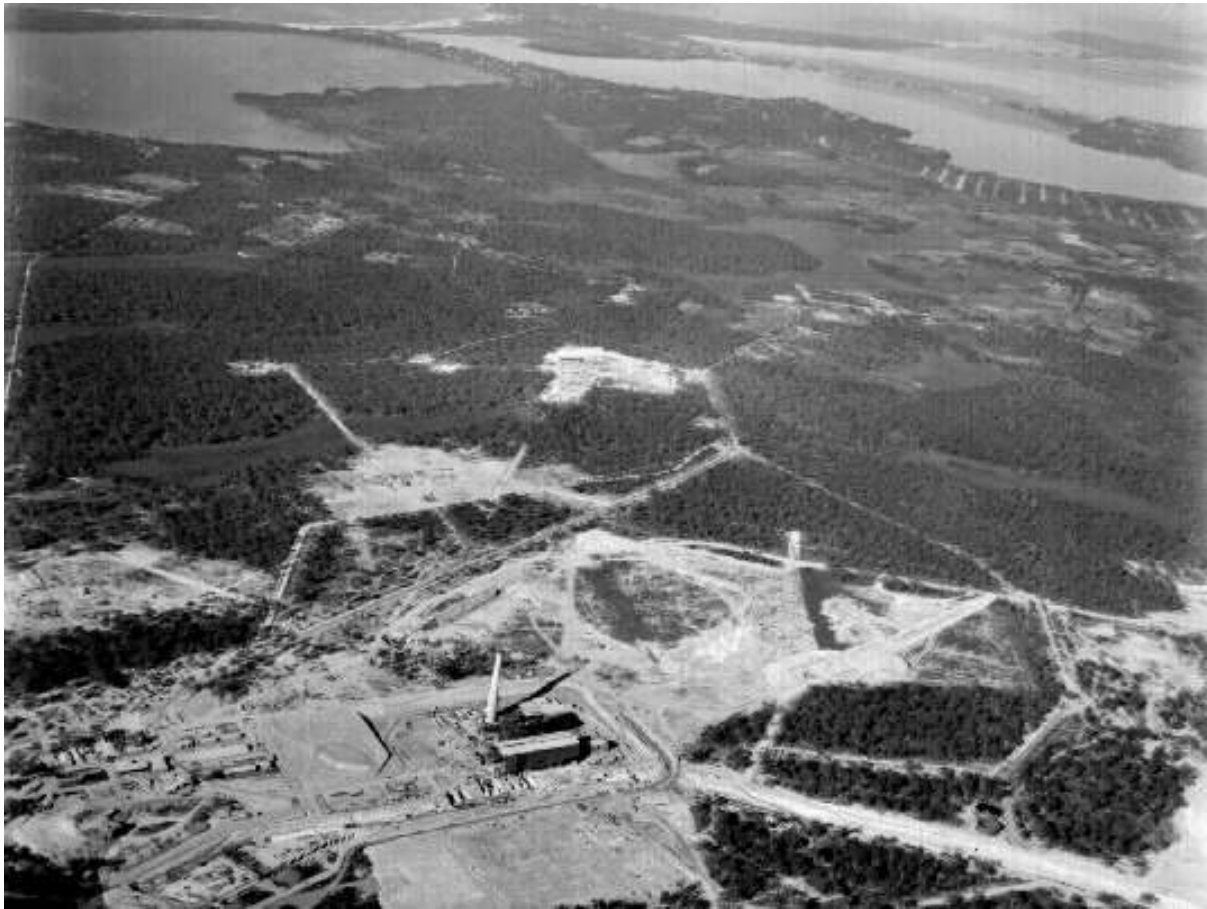
Vales Point Power Station, 1961.
