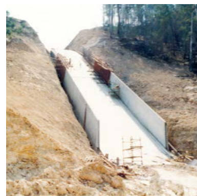
Construction of spillway bridge and spillway
