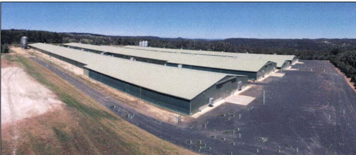
Figure 6: View of existing four sheds – fifth shed to be located at left in image
