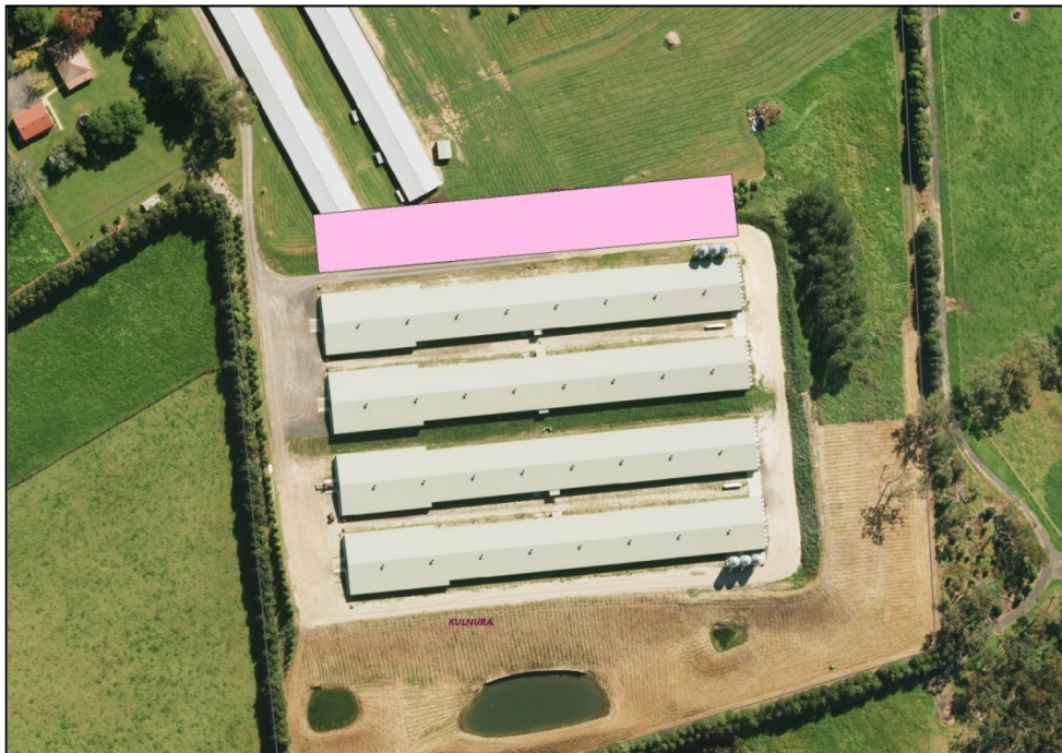
Figure 4: Aerial image with fifth shed approximately located in pink – note twin sheds at top of image have since been demolished.
