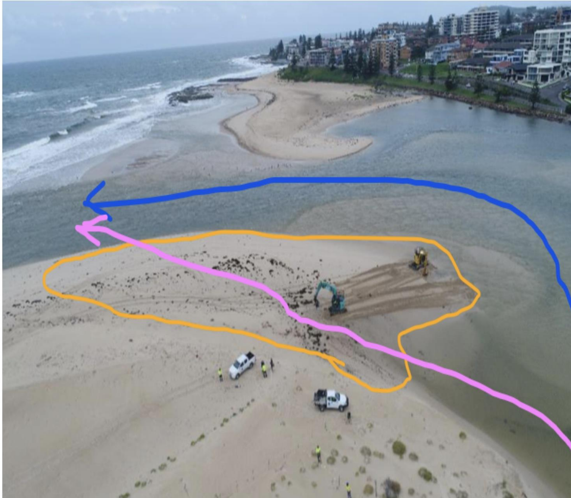
Figure 14: Channel Maintenance undertaken on Friday 19 March 2021 with approximate area of sand removal. The pre-existing general direction of 'ebb' channel flow is indicated with the blue line with sand removal works undertaken to allow for a more direct ebb flow channel as indicated by the pink line.
