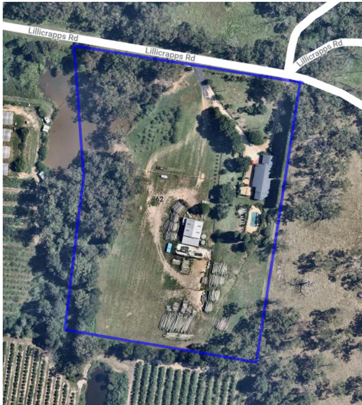
Figure 1 - Aerial photograph of the site 62 Lillicrapps Road, Mangrove Mountain
