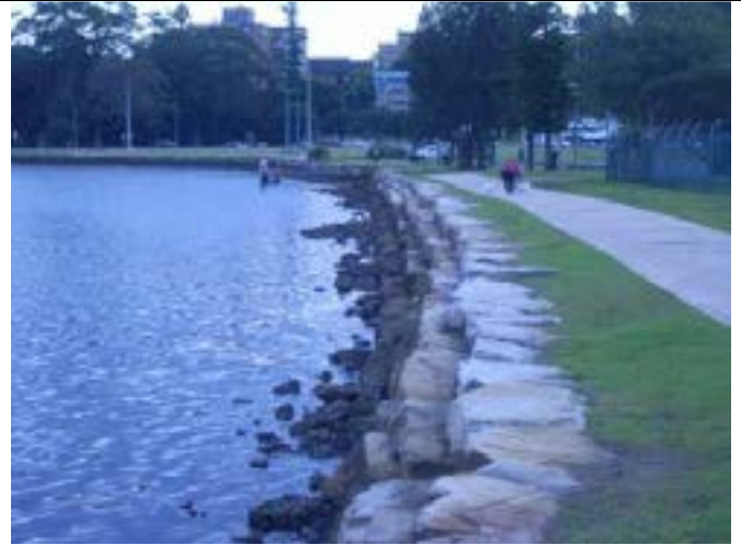
Photo 26: Point Frederick seawall looking north. (W69)
