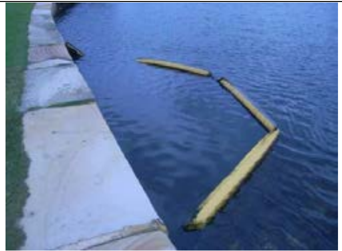
Photo 4: Stormwater traps along Gosford foreshore. (W27)
