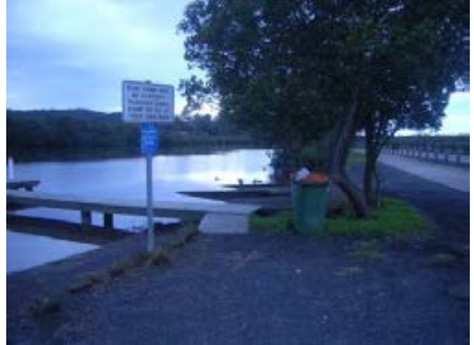
Photo 2: Boat ramp and jetty facilities at Erina Creek, looking upstream (north east). (W41, W107)
