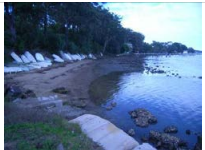
Photo 24: Informal dinghy storage along Masons Parade, Point Frederick (looking south). (W77, W86)
