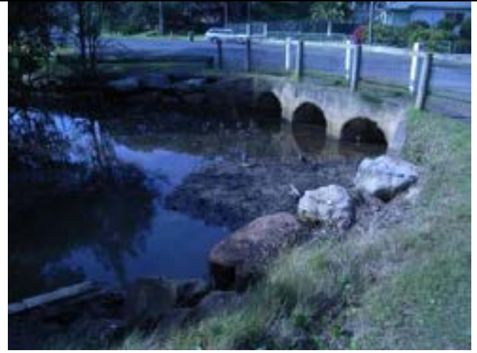
Photo 34: RSL Creek culvert into Hardys Bay. (W23)
