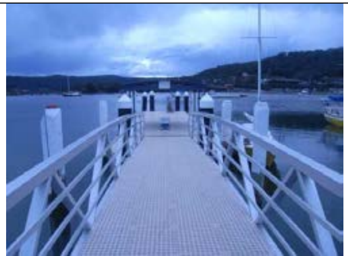
Photo 6: Gosford Public Wharf. (P48, R31)
