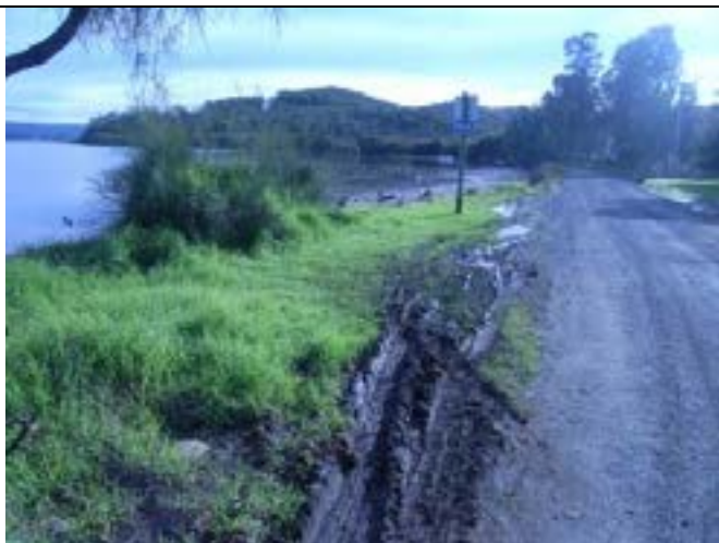
Photo 29: Looking north along Mundoora Avenue, Yattalunga. (W38,W63,W10)
