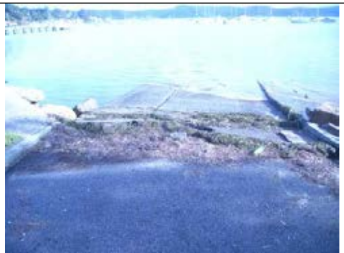
Photo 30: Centennial Avenue boat ramp at high tide. (W50, P48, R31)
