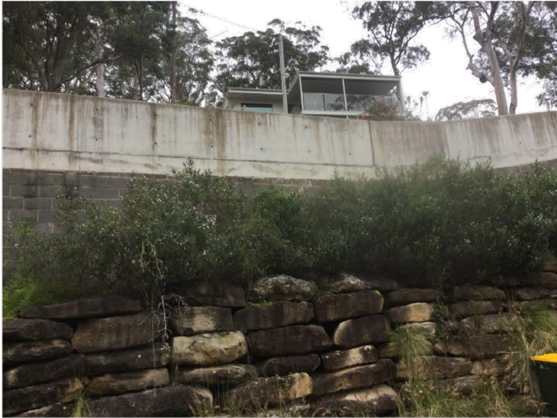
Photo 3 shows the retaining walls located on the high side of Fishermans Parade.
