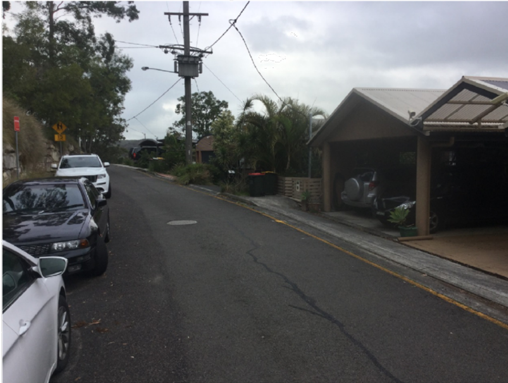
Photo 5 shows that car parking structures with reduced setbacks are an established feature of the street scape in the immediate vicinity.
