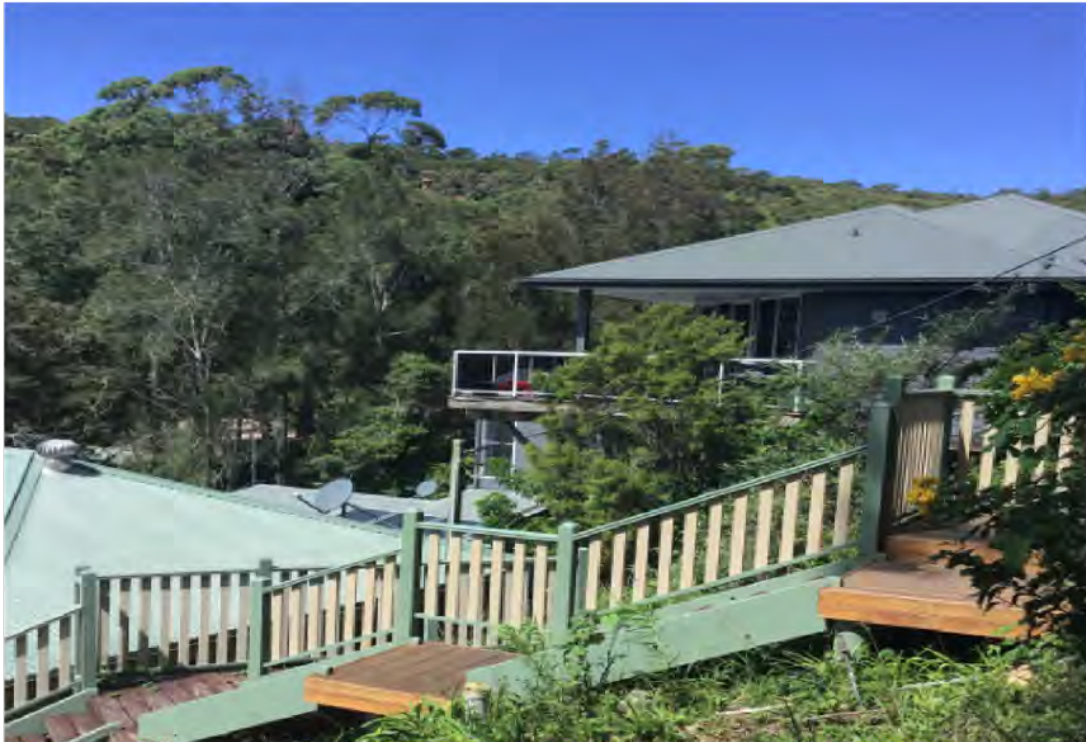
Photograph 2: Deck of No. 52 High View Road positioned above the ridge line of No. 50 High View Rd.
