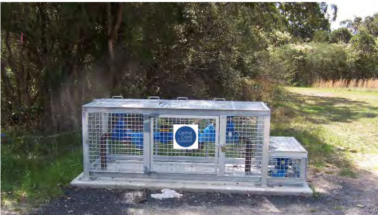
Figure 2: Example designated fill point for water carting at Wyee Road, Doyalson
