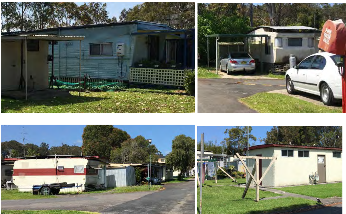
Above: Various photos of existing accommodation within the park (left and above) and amenities (right)
