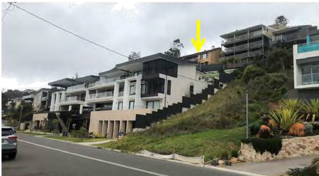
Photograph 2: Photos taken from public footpath along Avoca Drive. Subject site highlighted with yellow arrow. Note the four storey residential unit development downslope of the site.
