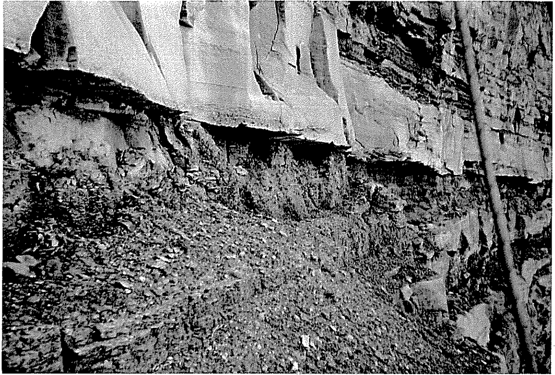
P.20. - SECTION 2. - WEATHERING OF UNIT D9 LOOKING NORTH.
