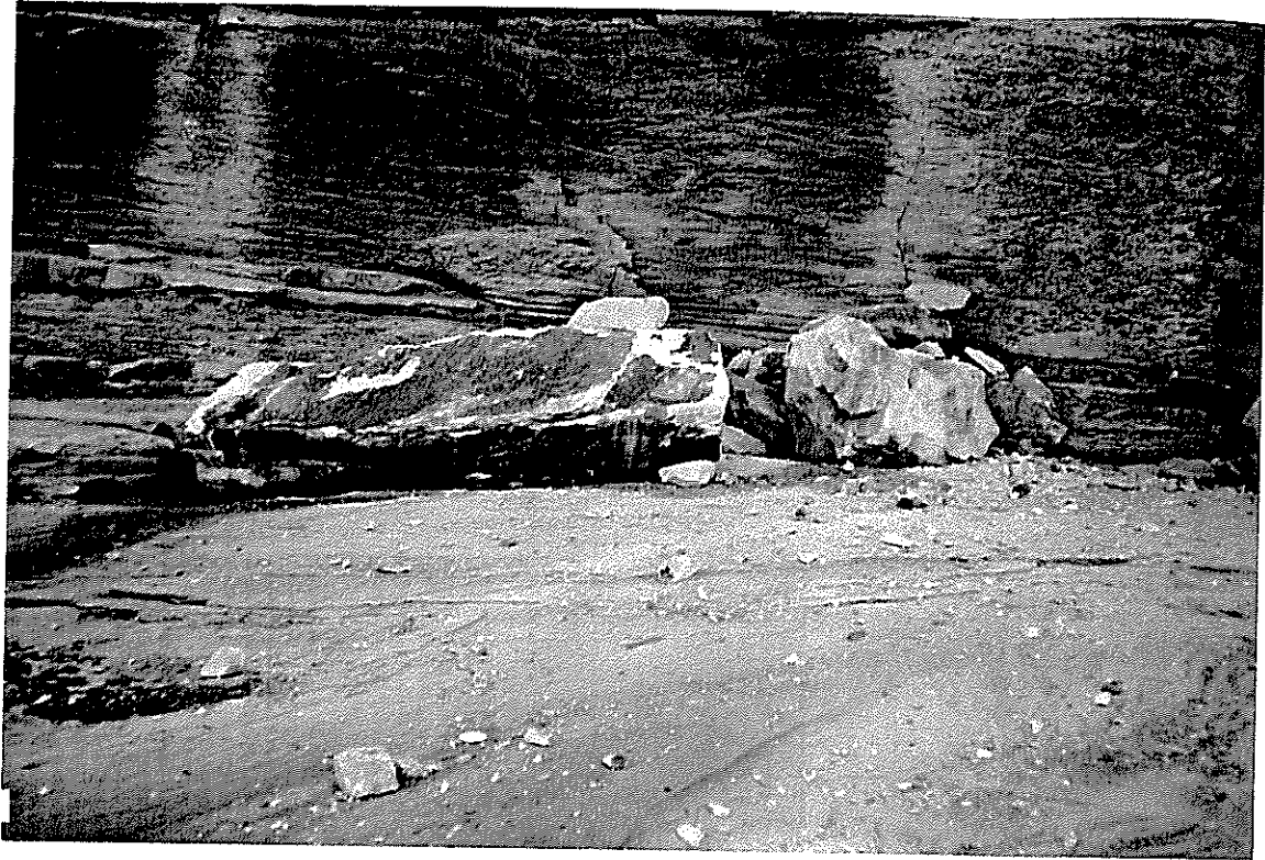
P.18. - VIEW OF ROCK DEBRIS FROM ROCK FALL NEAR LOT No. 876.
