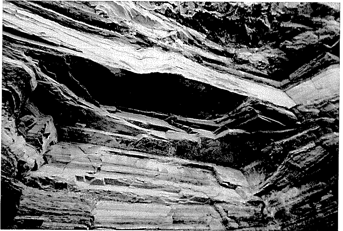
P.12. - STRESS RELIEF ROCK SPALLING IN ROOF OF SOUTHERN CAVERN.
