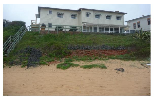
Figure 19: Rock basket and "seabee" protective works at 59-61 Ocean View Drive, 24 November 2011
