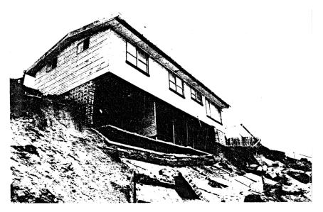
Figure 10: House severely damaged by dune erosion at Wamberal-Terrigal Beach in 1974 (from PWD, 1985)
