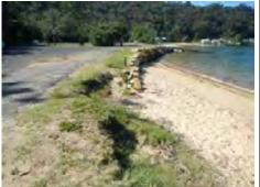
7. Existing erosion protection works at boat ramp and minor erosion adjacent to works
