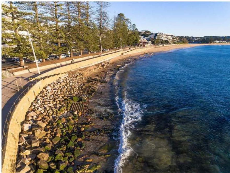
Plate 3 – Terrigal beach erosion and exposed former sea wall
