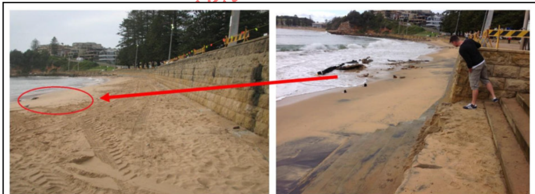
Plate 2 – 2016 Storm event at Terrigal Beach showing exposed timber sea wall and associated fill material.
