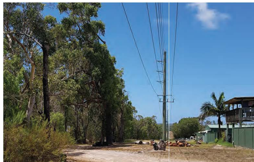
Figure 66: Electricity easement - Tall Timbers Road, Lake Munmorah
