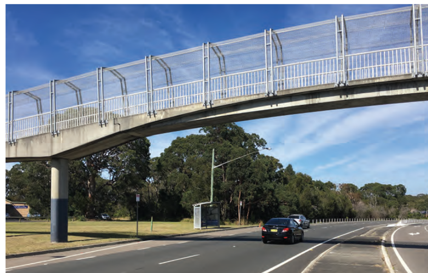
Figure 70: Pacific Highway overpass, Lake Munmorah
