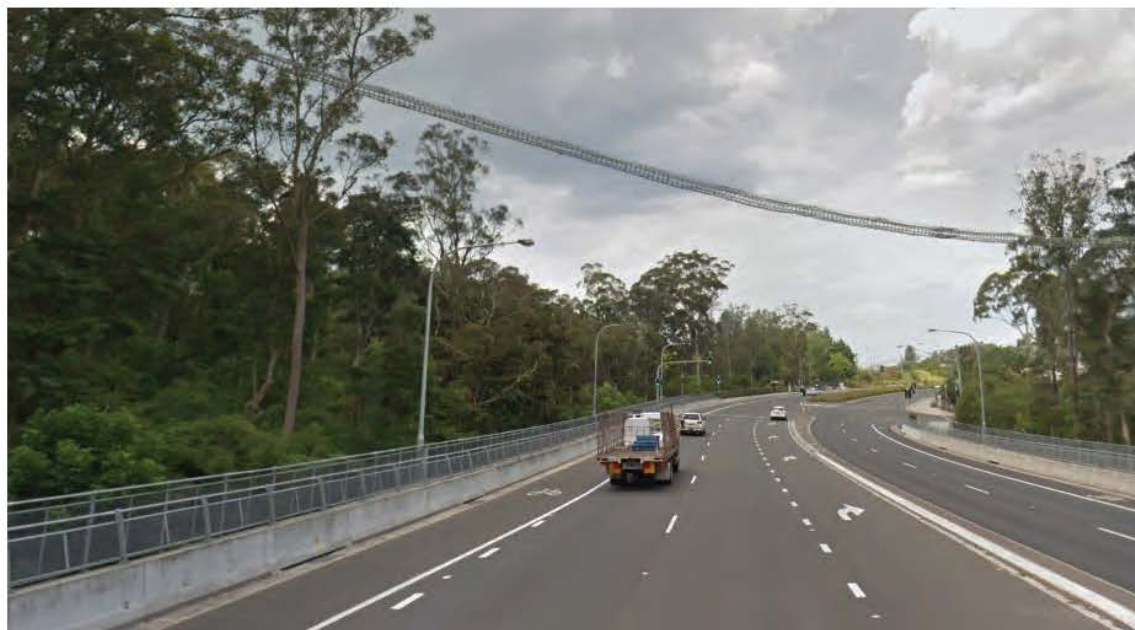
Figure 61: Aerial connectivity structure - Central Coast Highway, Wamberal
