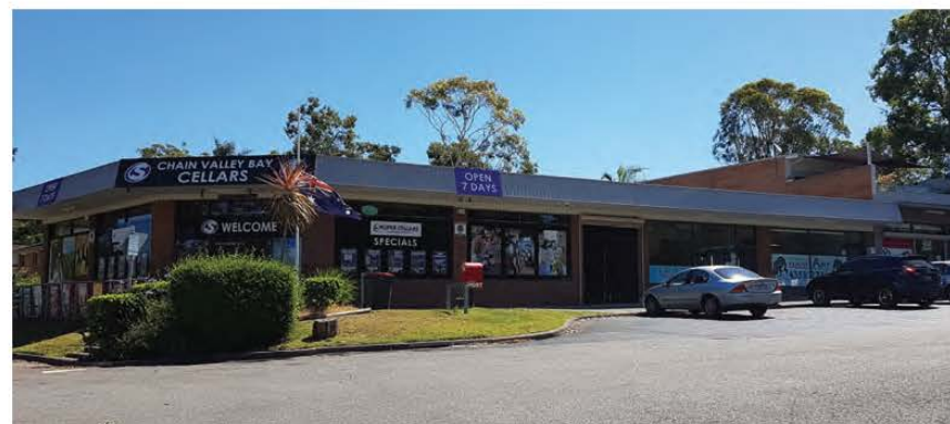
Figure 79: Chain Valley Bay Neighbourhood Centre
