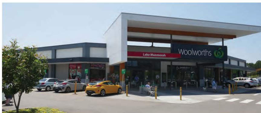
Figure 16: Existing Retail Centre at Tall Timbers Road, Lake Munmorah
