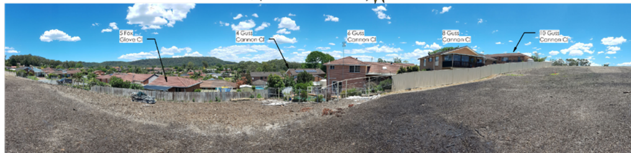
1 Panoramic view of subject site looking South West
