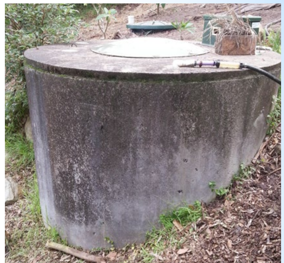
Above ground concrete tank
