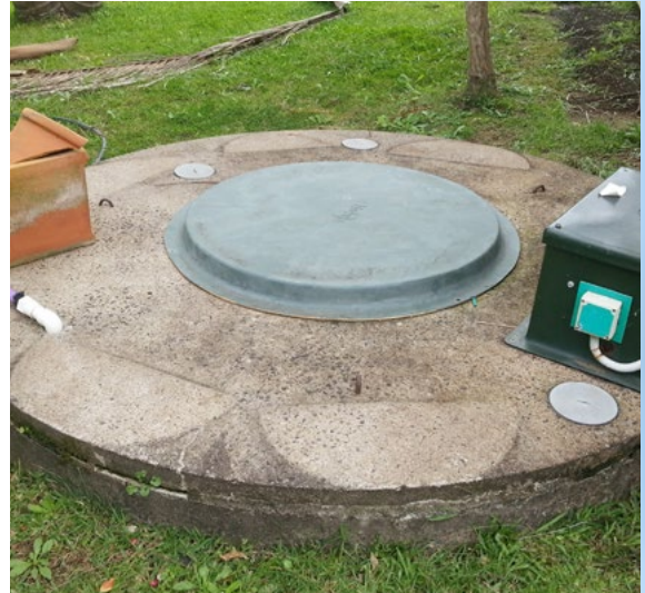
Below ground concrete tank
