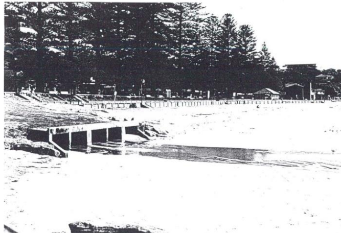
Figure 26: Existing Stormwater Outfall
