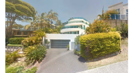
03. STREETSCAPE VIEW OF 46 CAMPBELL CRESCENT, TERRIGAL (SUBJECT SITE LEFT OF IMAGE).
