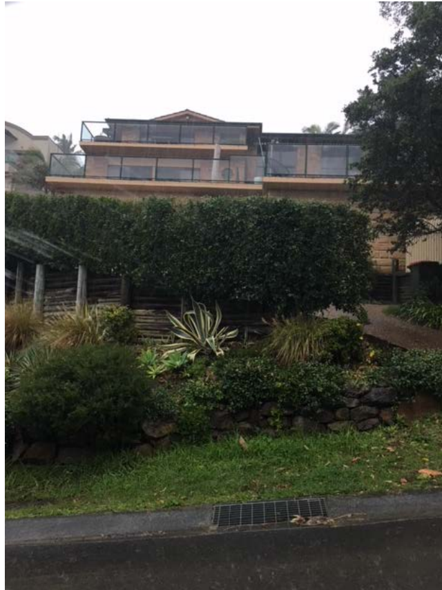
Figure 5 – View of adjoining property to south, No. 42 Campbell Crescent
