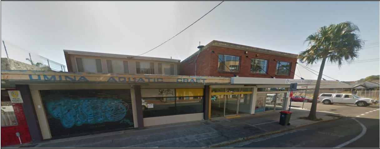
Figure 2 – West Street frontage of the site
