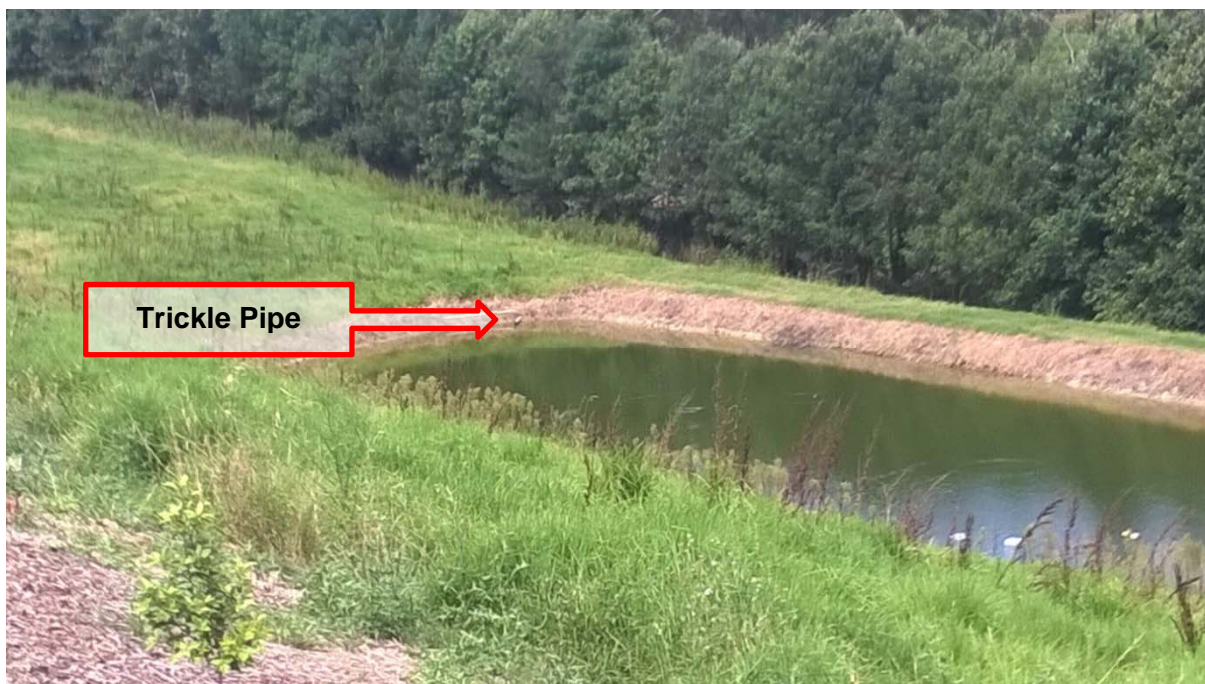
Figure 13: Dam to the south of the existing poultry sheds on the subject site (trickle pipe visible on the bank of the dam above water level)
