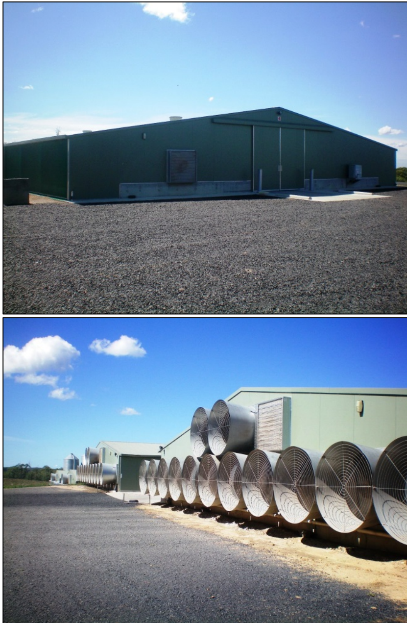
Figure 2: Front (left image) and rear (right image) of existing tunnel ventilated poultry sheds
