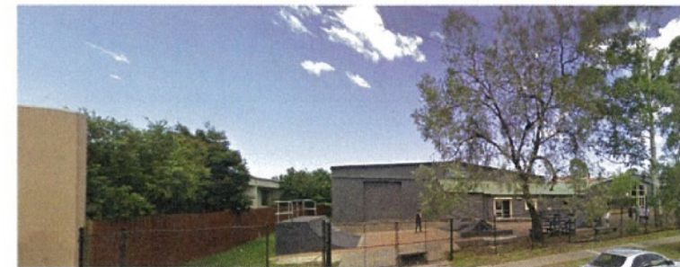
View from North West Corner
