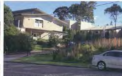
FRONT ENTRANCE OF ANGLICARE NORTH WEST TOWARD FROM SOUTH SIDE OF MATARAM ROAD
