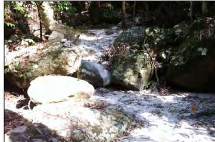
Sugarloaf Conservation area – Failed attempt to remediate subsidence induced surface cracking
