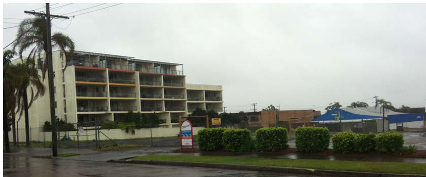
Above: Residential building located at Warrigal Street facing new loading dock
