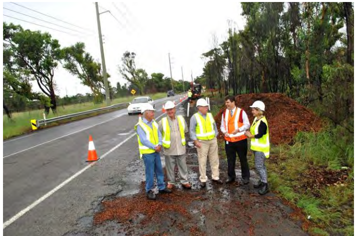
Ruttley's Road works on target
