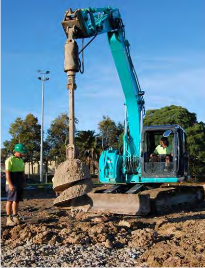
Levelling the site for the Metro Cinema
