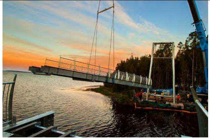
Ten storey crane places sections of the bridge at Berkeley Vale
