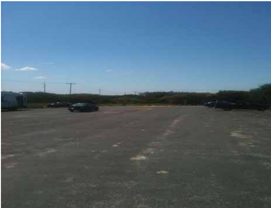
View Carpark north of site 1
