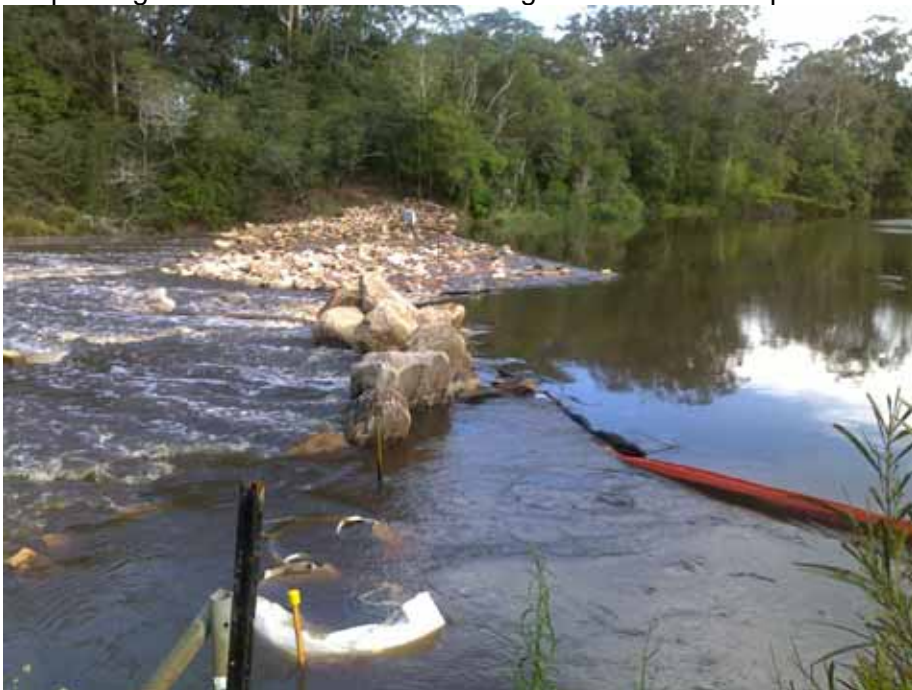
Construction of the fishway on Wyong River (Work Package 18)
