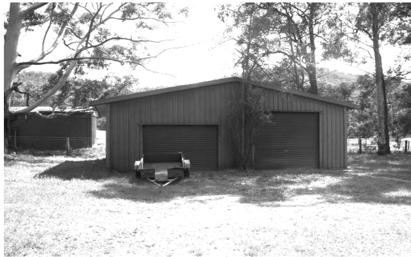
Figure 1: Existing shed to be used for boarding kennels.
