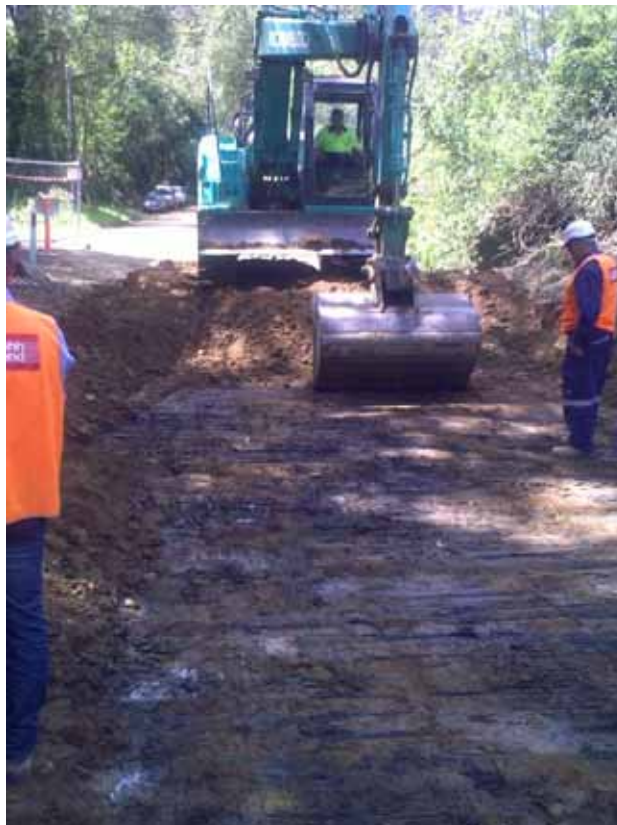
Discovery of corduroy road at Kidmans Lane.
