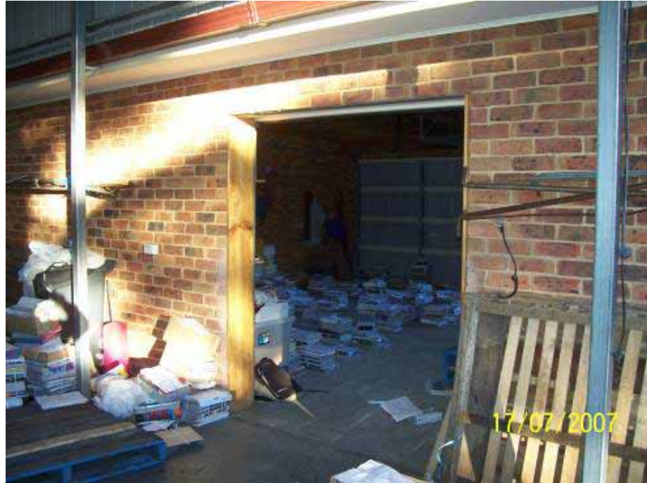
Figure 3: Interior of triple garage
