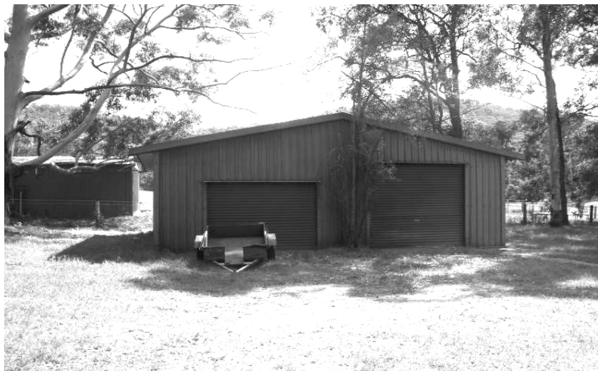
Figure 1: Existing shed to be used for boarding kennels.
