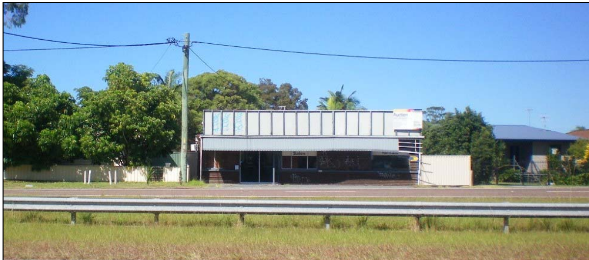
Figure 1. Site as viewed from the Pacific Highway
