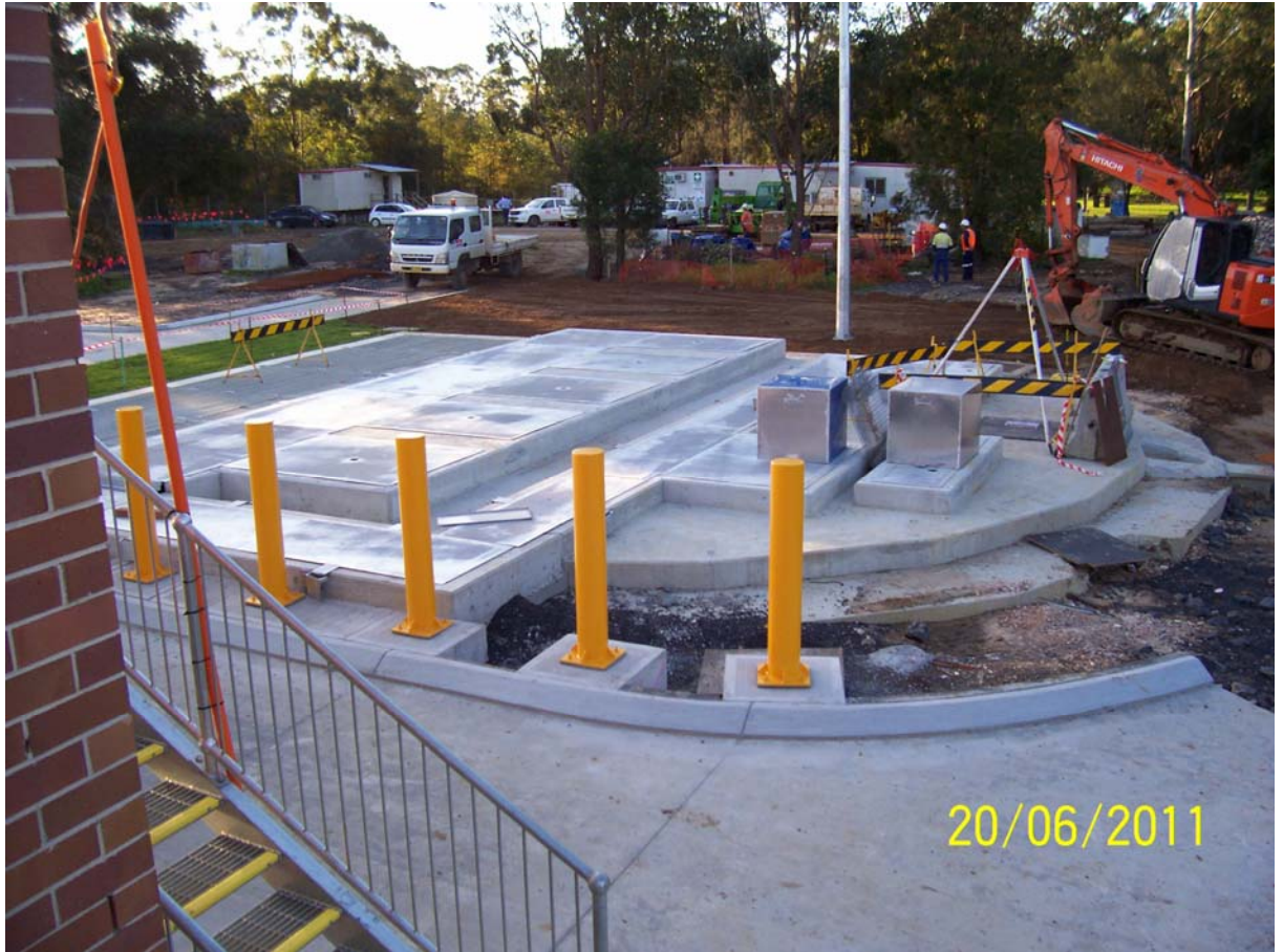
Installation of the pump station wet well lids. (Work Package 2)
