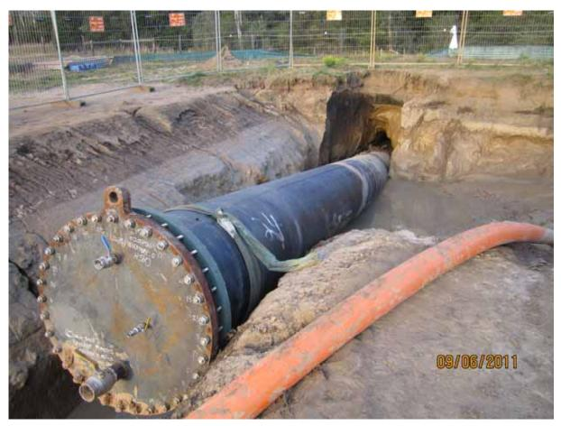
The installation of the 260m HDD pipework has now been completed. (Work Package 7)
