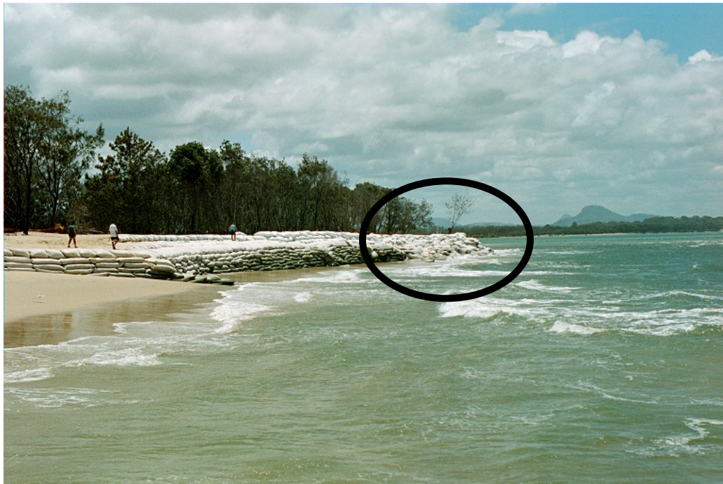
35m rubble section
