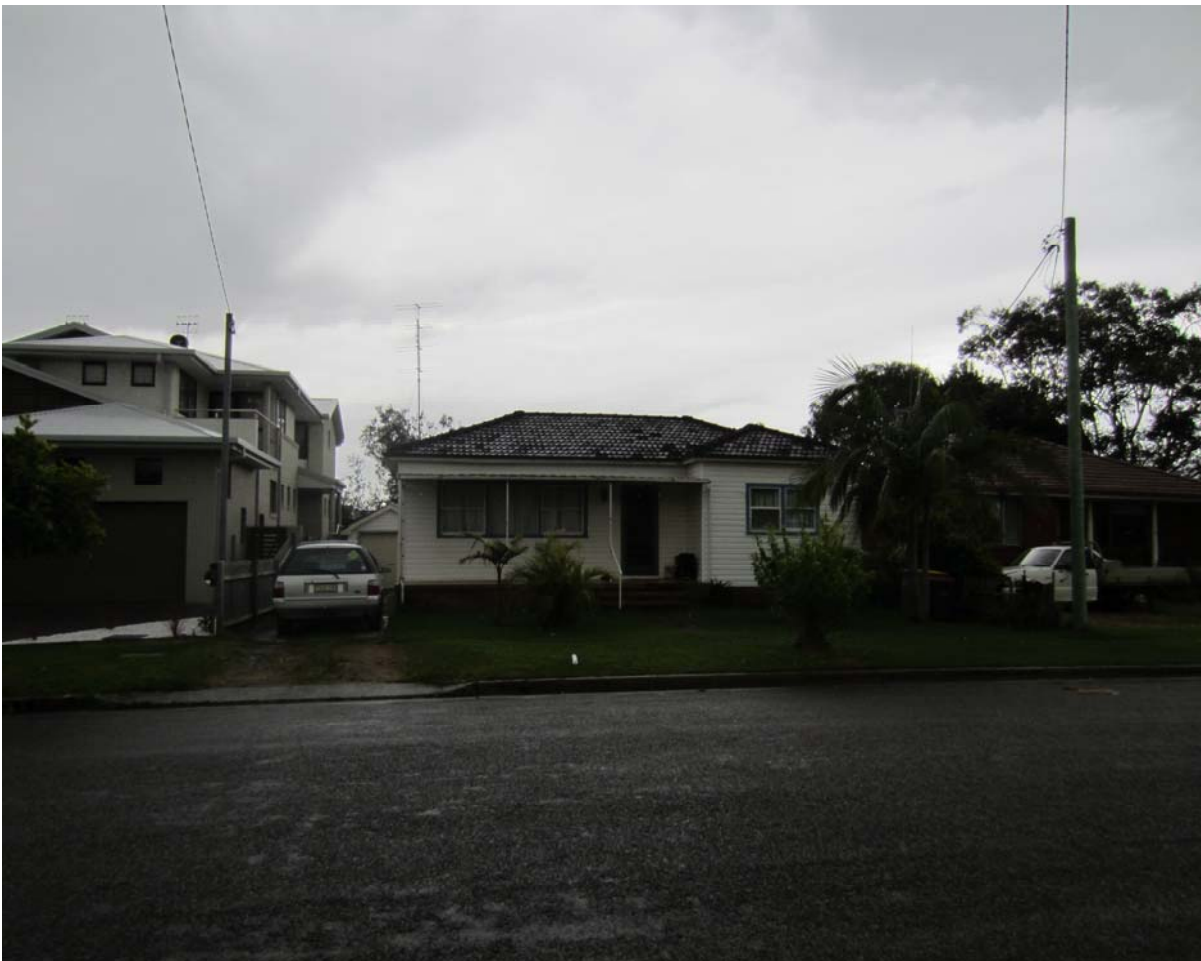
The proposed site and existing timber clad dwelling that is proposed to be demolished
