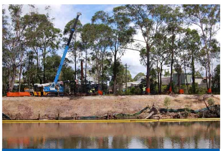
Works are underway to stabilise a section of the bank along Ourimbah Creek as part of the Tuggerah Lakes Estuary Management Plan. Ourimbah Creek is one of five tributaries that flow into the Tuggerah Lakes that are having restoration works carried out and aim to improve water quality of the Tuggerah Lakes.
