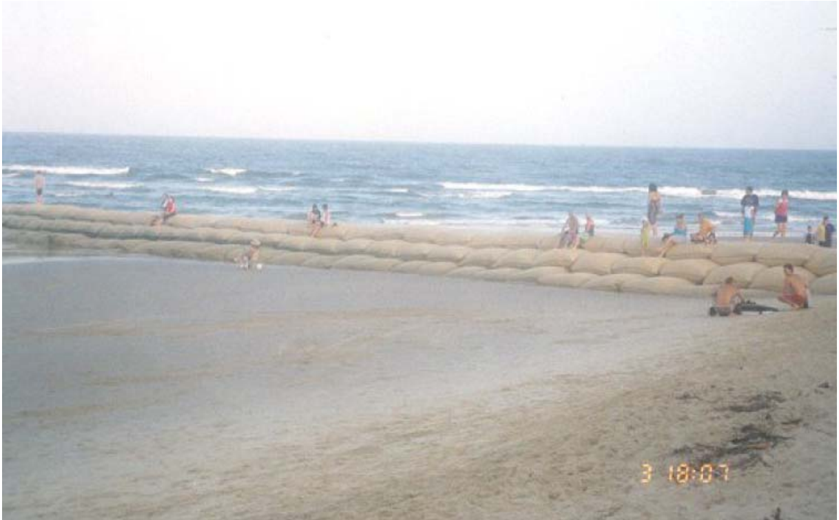
Source: Detailed Conceptual Design of Beach Bore Intakes and Brine Discharge to Ocean – Temporary Desalination Plants, Wyong Area, WRL, 2006
