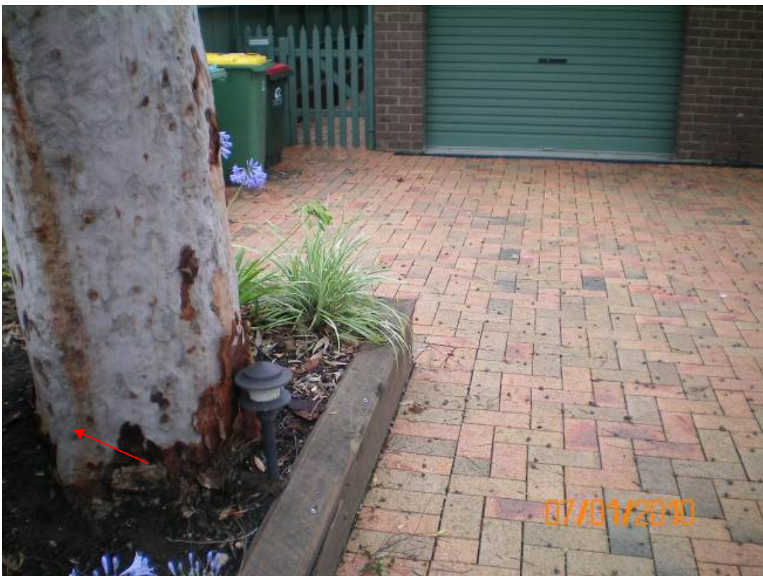
Brick paving appears unaffected by tree roots.
