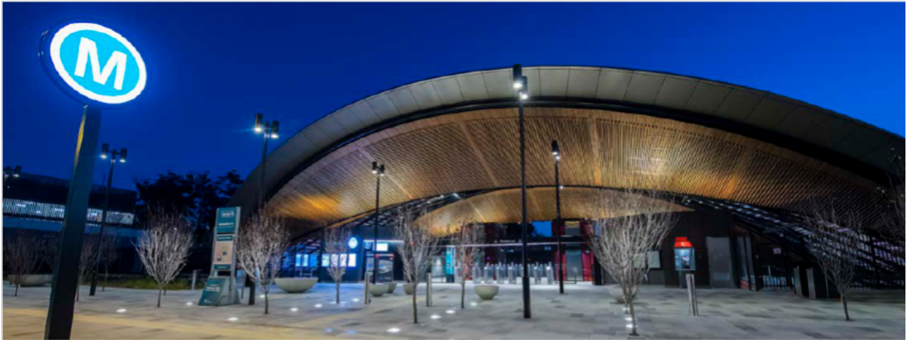
CHERRYBROOK METRO STATION Photo credit: Sydney Metro
