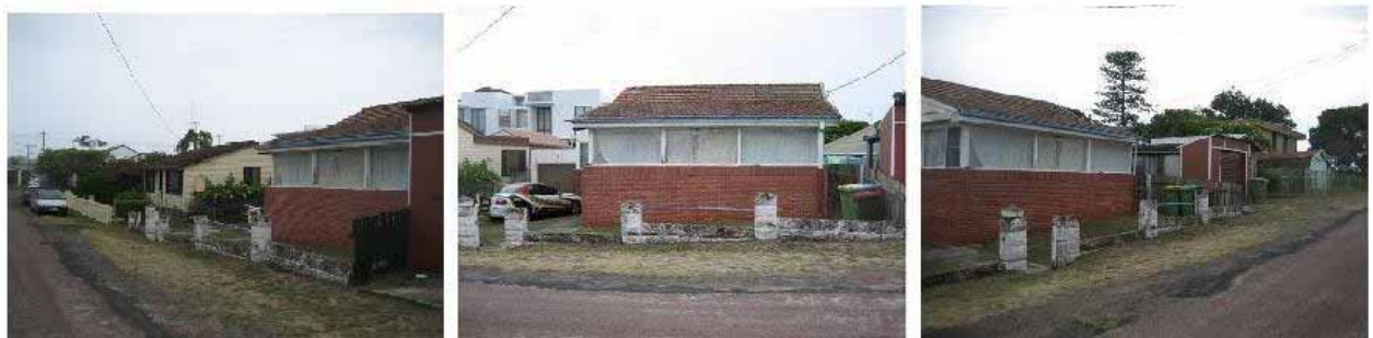
Brogden Road streetscape with the recently completed residential flat building in the centre background
