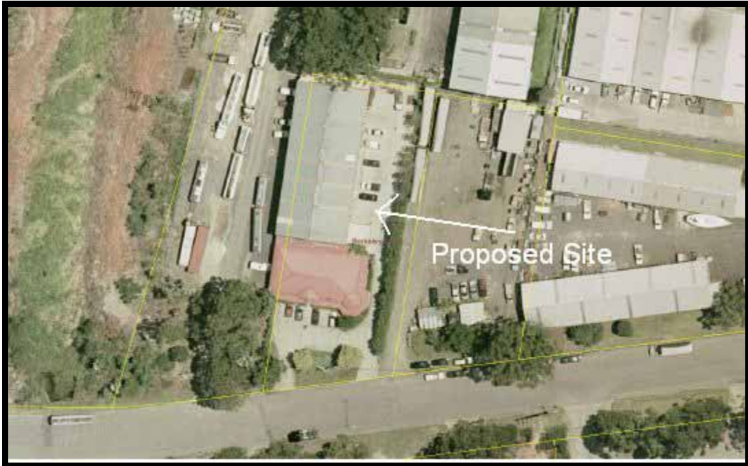
Figure 1: Aerial photograph of the site.
