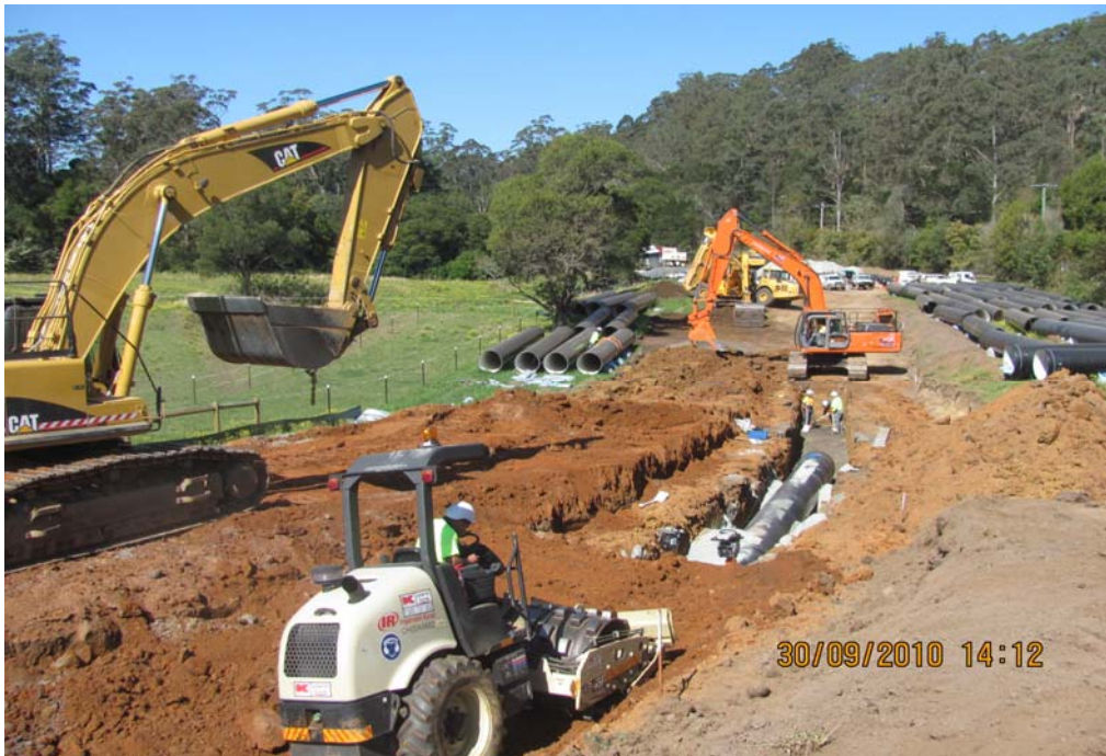
Typical Pipeline Laying
