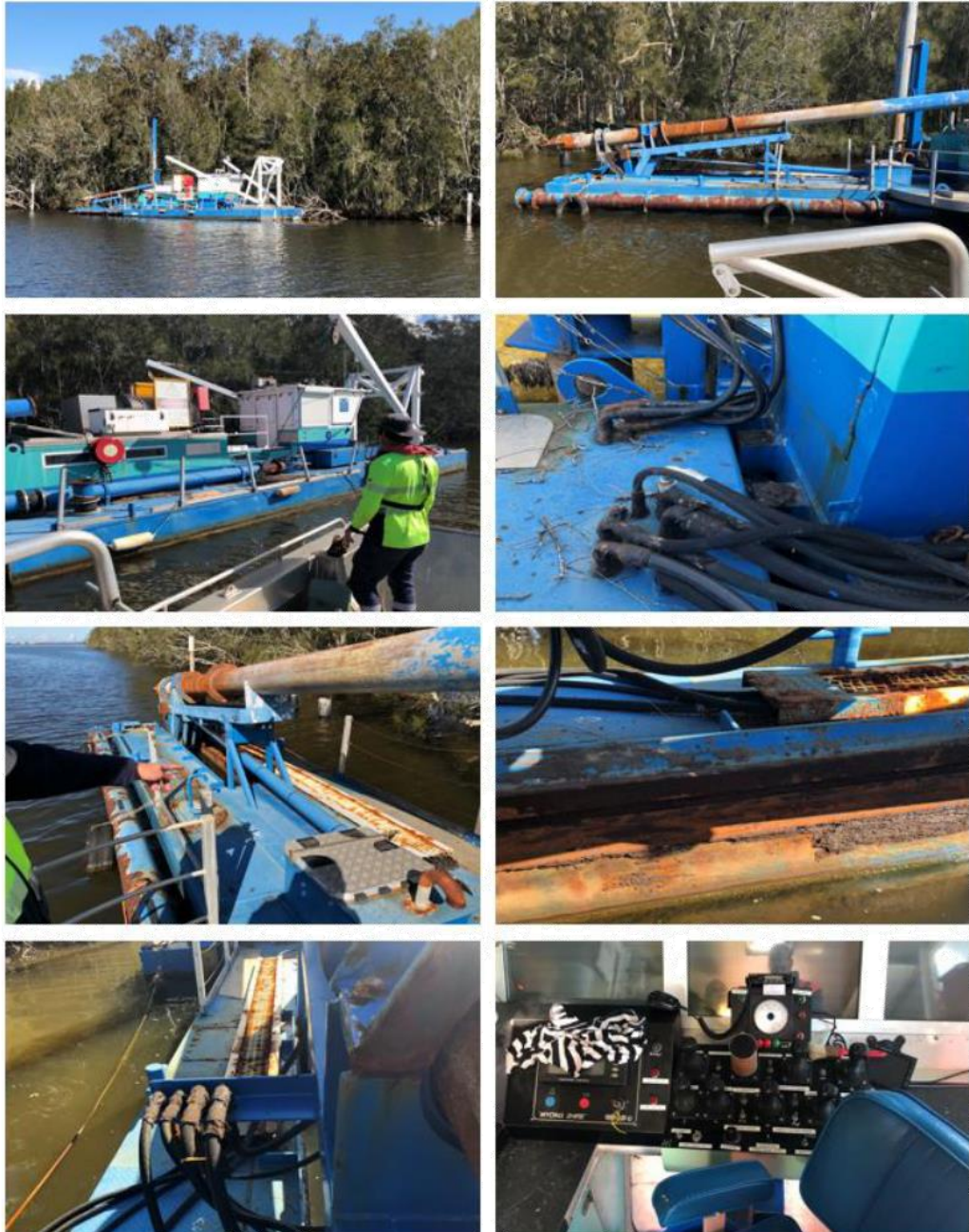
Figure 4-2 Council's existing dredge photos 16/05/19
