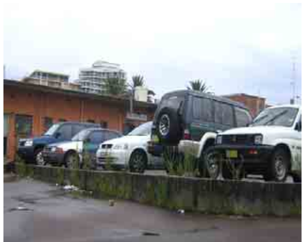
Fig 5.6.6 Looking at the front of the Car Park (Source: Dickson Rothschild)
