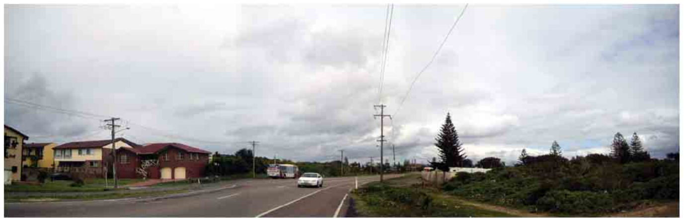
Fig 5.1.6 The Entrance Road near Hutton Road present condition
